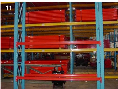
Additional rack bays and beam levels may be added as shown in photograph 11. The rack unit, shown in photograph 12, is now completed and Row Spacers, if desired, may be installed. Row Spacers are used to space rack rows placed back to back. They also act in distributing forces should the rack be struck. Row Spacers should always be installed in line with, or near a Horizontal Truss member.
