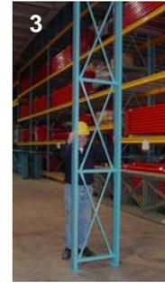
Photographs 1, 2 and 3 show a Truss being raised to its upright position. Make certain the Truss Base does not slide by placing a foot on the Bottom Horizontal brace.
