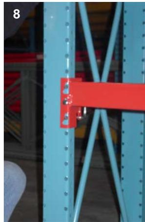
While steadying the Upright Truss with the Beam connected and locked in place, raise another Truss and connect the Beam as previously outlined, and as shown in photographs 9 and 10. Continue working in one direction setting up rack bays. Do not set up bays from two ends working toward a center.
